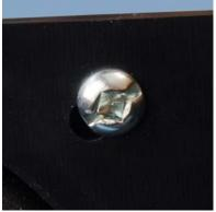
The screws must not be over torqued, or the plastic plate may crack.
